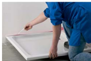
3. Remove upper protection foil.
