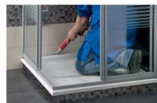
6. Apply silicone joint.
